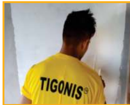
WALL PUTTY APPLICATION
