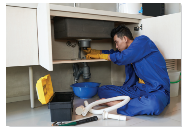
Wash basin/Sink plumbing work
